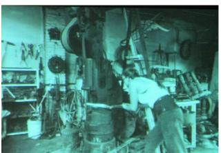
metal is shaped by hammering. The forge is a device to hold a fire for the purpose of heating metal for shaping. The post vise (strapped to a support post) holds firmly hot iron while it is hammered.
