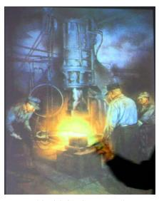
Tongs are used to grasp and hold the hot metal.
