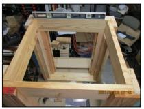
The modifications I made to add wheels to the table included shortening the length of the inner 2x4 legs. To ensure equal space to accommodate the 2x6 support for the wheels I flipped the table to assemble it upside down. I figured gravity would help me with the spacing. I rested the 2x4 inner legs against the 2x6 supports flush with the top of the 2x6 legs. I then attached the inner 2x4 legs to the outer 2x6 legs. A 2x6 is attached between two pairs of legs.
